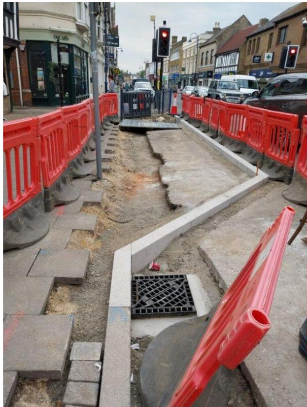
**07/05/2024 – New kerbline laid at Church St pedestrian crossing prior to new slot drain installation and slab laying.**
