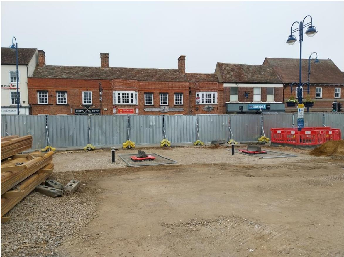
**07/05/2024 – Completed rain garden system installation after backfilling. Holes covered in preparation for tree planting.**
