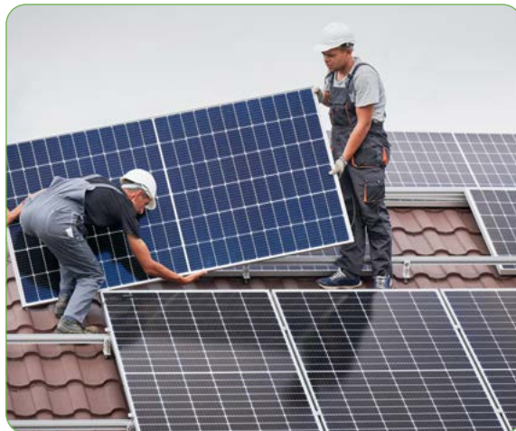
Technicians installing photovoltaic solar modules on the roof of a house
