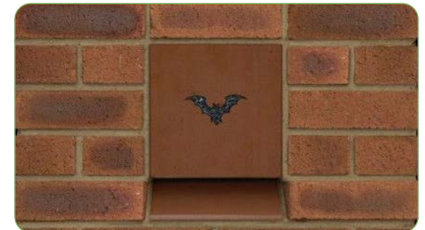
Bat Box built into a wall
