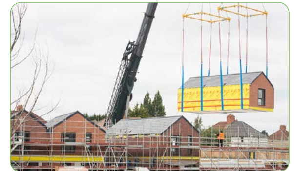
Modular homes being lifted into place on site (source: www.constructionnews.co.uk )
