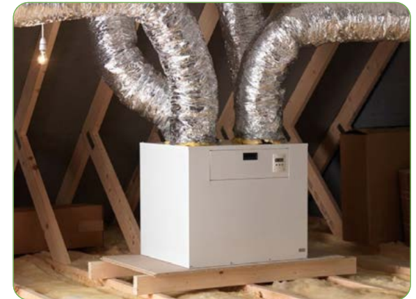
Typical domestic MVHR system fitted in the roof space (source: https://sgs-energy.co.uk ).
