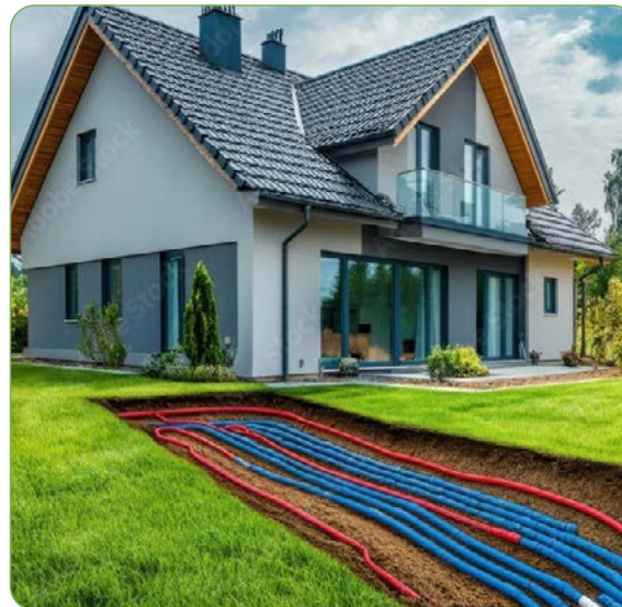
Pipe loop serving a Ground Source Heat Pump
