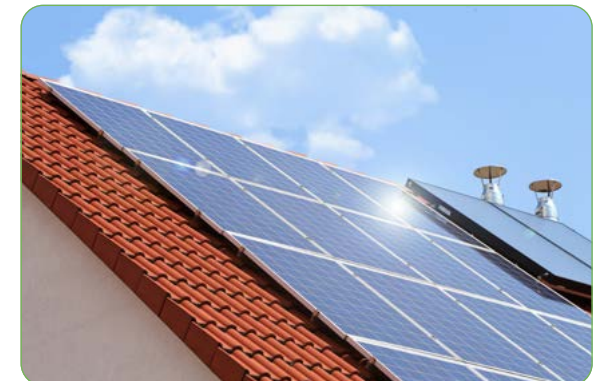
PV panels that have been retrofitted to the dwelling and sit proud of the roof tiles
