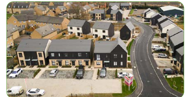
California Meadows, Huntingdon - development used timber framed panels manufactured in factory conditions before being transported to site and craned into place (source: www.longhurst-group.org.uk )
