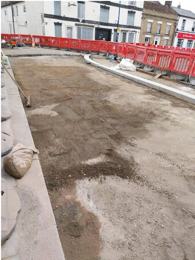
*17/07/24 – New kerb line installed and next section of Market Place stripped back and graded ready for block laying*
