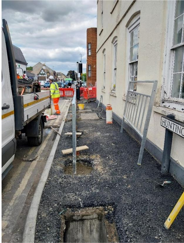
*17/07/24 – New pedestrian guard rail being installed at Huntingdon Street crossroads ready for surface tarmac course to be laid.*
