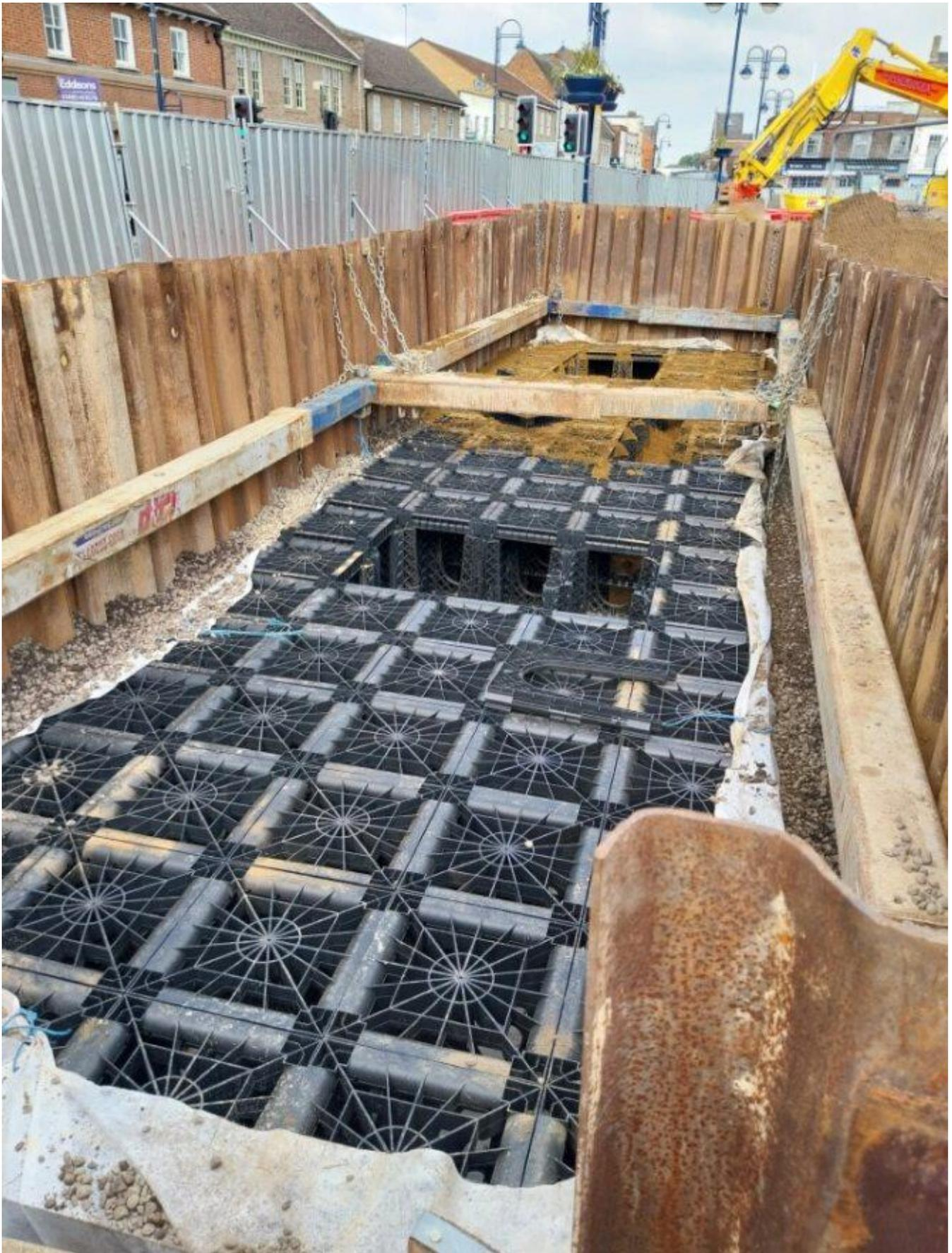
***01/05/2024 - Installation of rain garden planting system in NW corner of Market Square and backfilling.***
