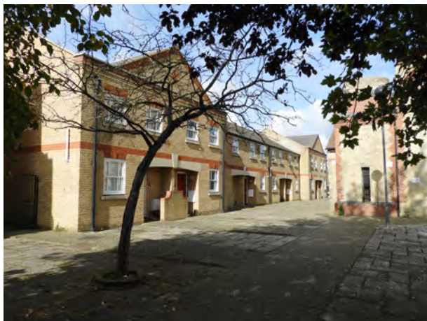
Modern infill development can blend sympathetically within a historic environment as achieved in homes adjoining Paines Mill
