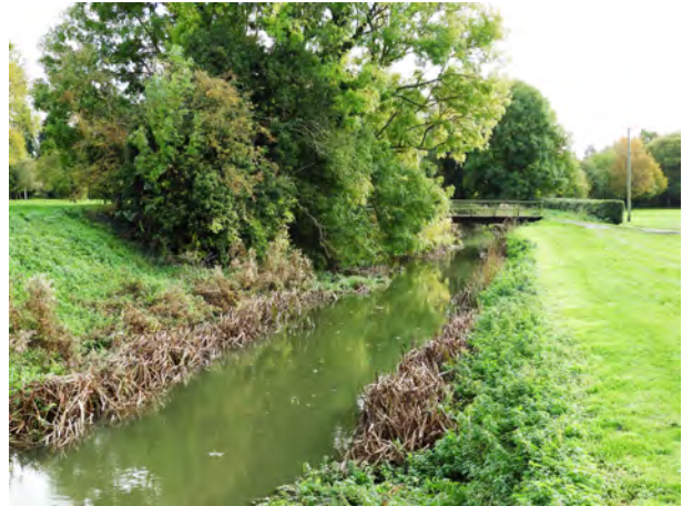
High Lode watercourse flows through the whole area surrounded by open space
