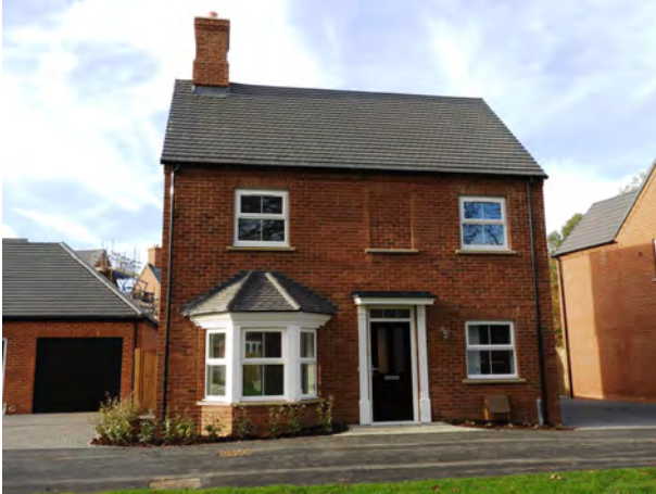
Development of new homes on the former RAF Upwood clinic started in 2019
