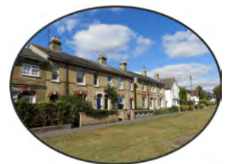
Terraced homes facing onto the park
