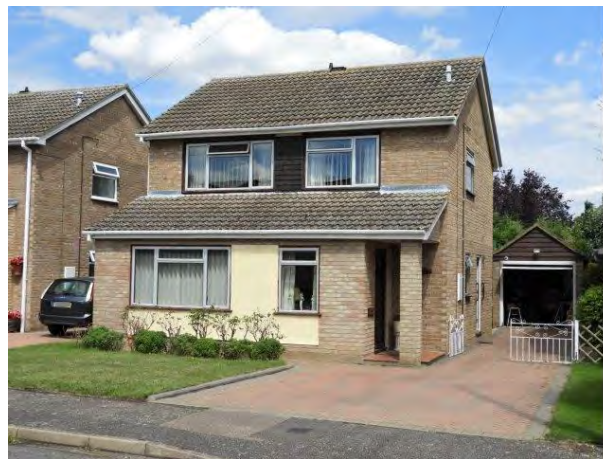
Pale brick homes with large windows and tile hung detailing are widespread in this area
