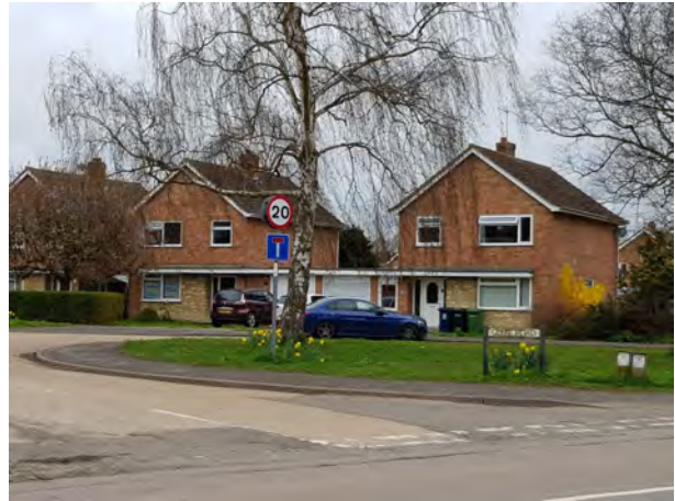
Two storey properties within Glebe Road with connecting flat roof garages and open space to the front where Glebe Road connects to Church Road.
