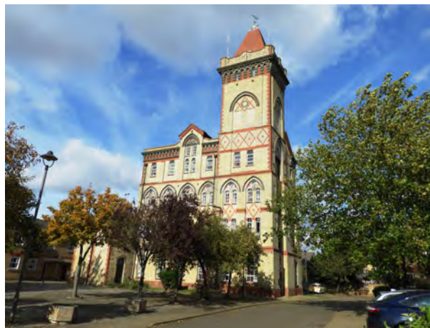
The elaborate brickwork and height of Paines Mill tower form a highly distinctive local landmark
