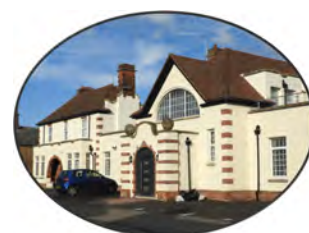
Converted Police Station on Blenheim Road
