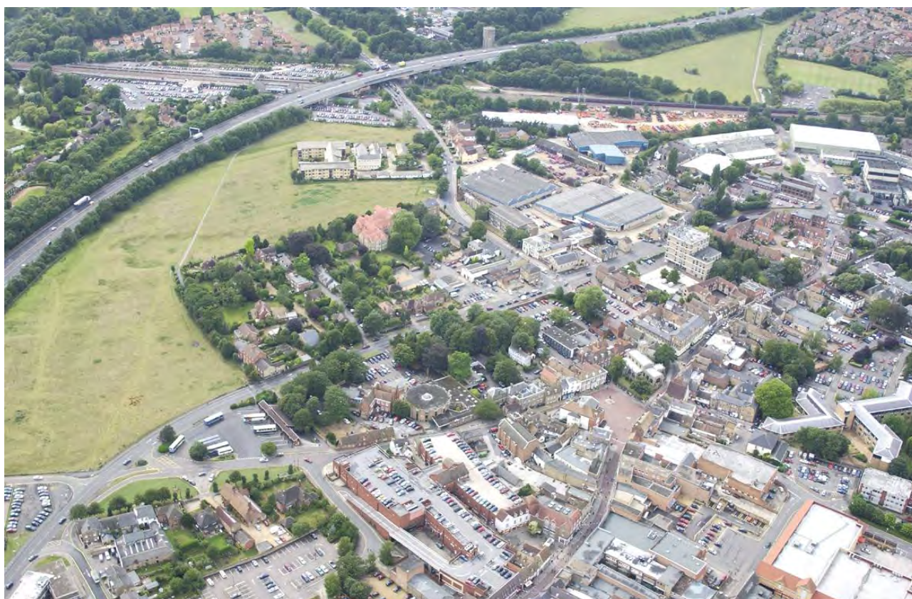
The A14 trunk road as it passes around the south western edge of Huntingdon town centre.
