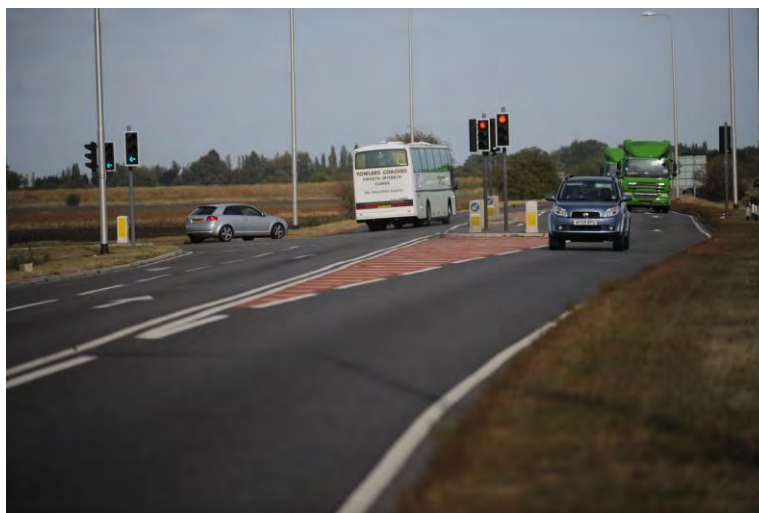
The Goosetree junction of the A141 between March and Wisbech, and the A605 to Whittlesey
