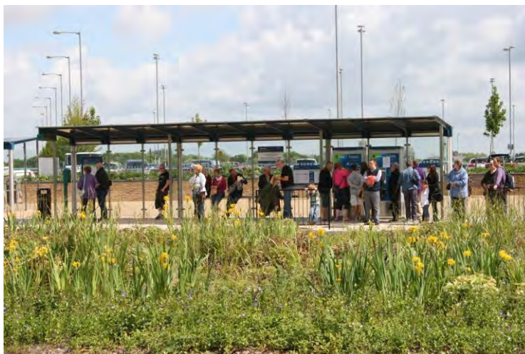
The Busway at the St Ives Park and Ride site
