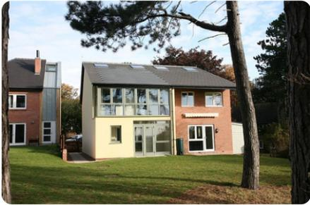
4.6.12 The other key difference in the two homes is the energy supply. The level-six home needs to be totally self-sufficient. The electrical load for the house was calculated at 3.5kWh and on the south-facing roof 22m<sup>2</sup> of photovoltaic (PV) tiles with a peak generating capacity of 3.7kW were installed. This is what drove the asymmetric roof design as it is the only way they could get the area of PVs needed. The integrated tiles were seen as the neatest solution.
