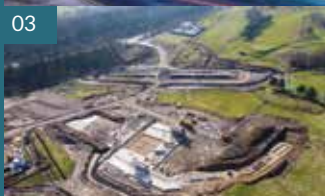
01. NDA Archive, Caithness 02. 40 Brighton Road, Surrey 03. Skipton Flood Alleviation Scheme, Yorkshire
