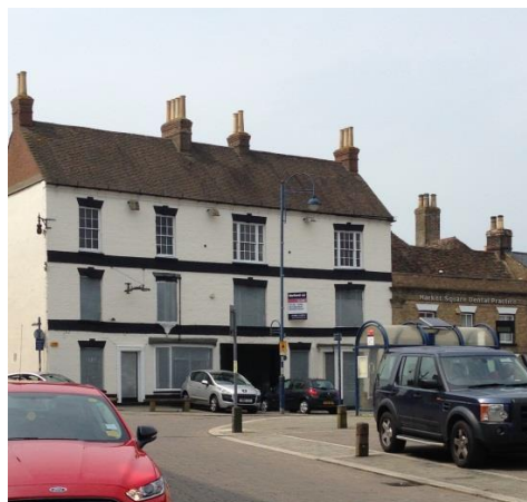
Figure 4.18: The old public house at 10-12 Market Square has been vacant for a number of years.
