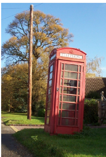
Opportunity for enhancement - The listed Telephone Box on Easton Road is need of maintenance.
