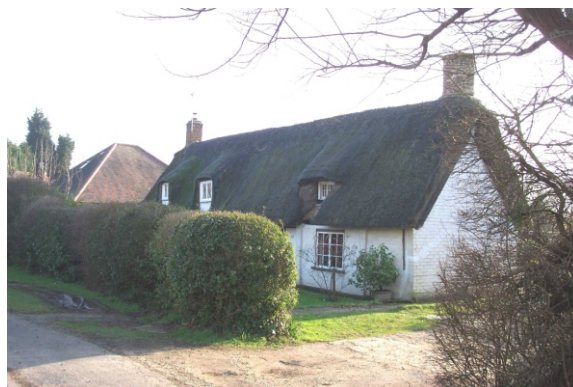
April Cottage dates to the 17th century and is a one and a half storey dwelling with dormer windows.
