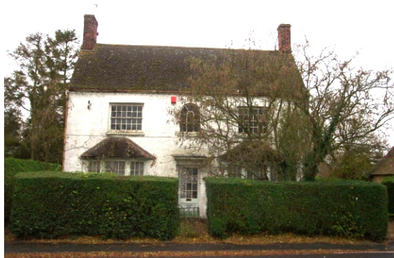
Opportunity for enhancement- Stonely House has been vacant since 1970s and would benefit from repair.
