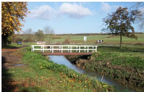
The river Kym appears as a gentle stream, in summer, as it passes under the pedestrian bridge situated at Stonely Green.
