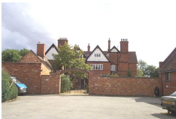
Opportunity for enhancement - the approach to Stonely Grange detracts from the setting of the house. Improvements to the parking area and to the way parking bays are defined would enhance this area.
