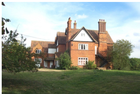
Stonely Grange along with associated stable block dates to 1864-65 and is built in the Vernacular Revival Style. The architect was John Devey, who was nationally acclaimed in his day.
