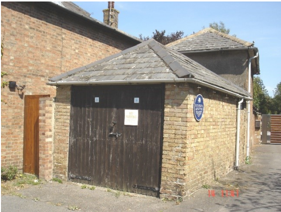
Fire Pump Accommodation
