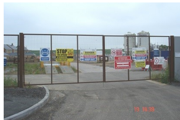
295 Bovis Homes under construction in 2022
