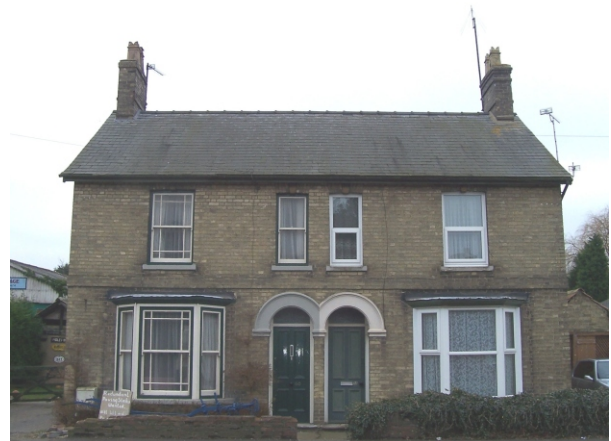
A building typical of Warboys in form and details, built in the style of the detached villas, but in this case a pair of houses without the usual green frontage. The replacement windows of the property on the right-hand side alters the character of the building and detracts from the conservation area.
