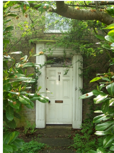
Front door to 26 High Street
