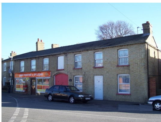
Local shop on the pavement edge at the start of the High Street, by the clock tower. Modern signs and replacement glazing have somewhat disrupted the appearance of this building
