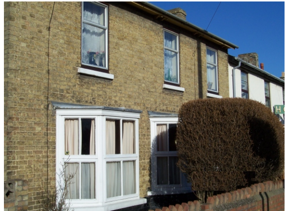
This particular property has two different styles of replacement window, one to each floor.
